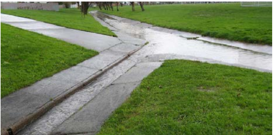
Fig. 1 Concrete channel confluence, Naenae Park
