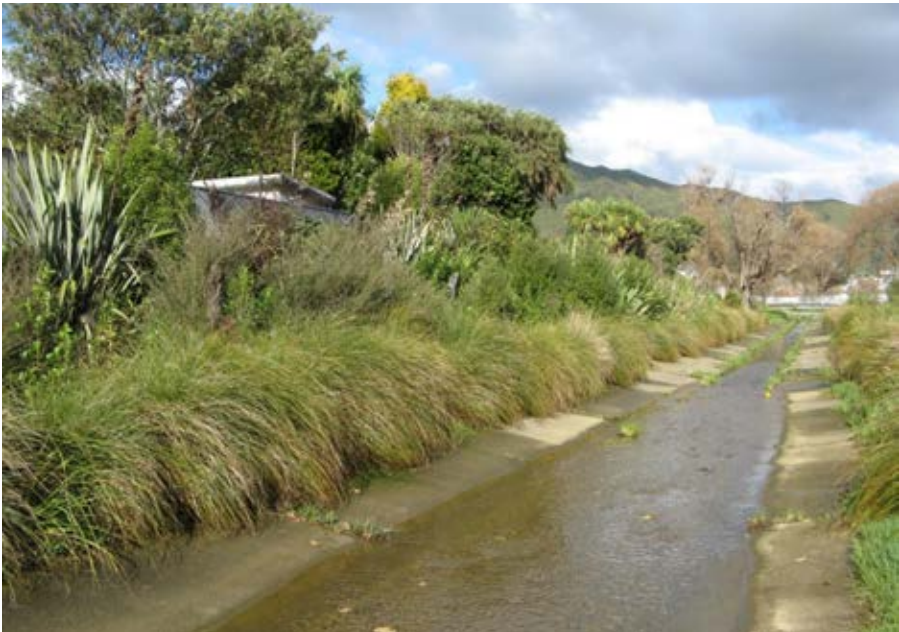
Fig. 9 Carex secta draping over edge of concrete berm and taller plantings at the back
