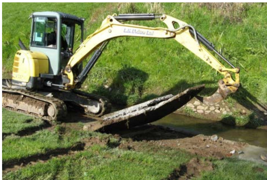
Fig. 2 Digger removing concrete berm
