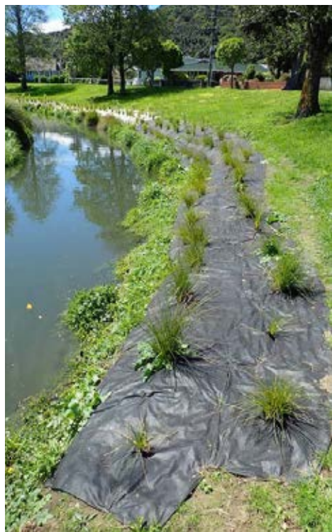
Fig. 1 Non-woven polypropylene as part of the trial. Image: Chris Cosslett
