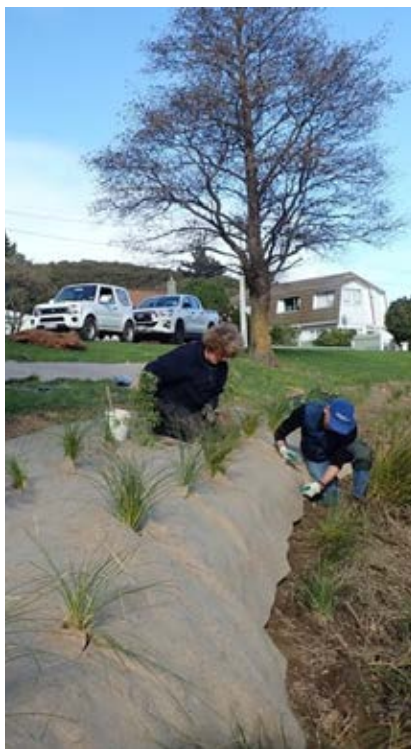
Fig. 2 Laying ecojute. Image: Chris Cosslett.
