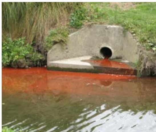
Fig. 1 Paint pollution through a stormwater pipe from a residential property
