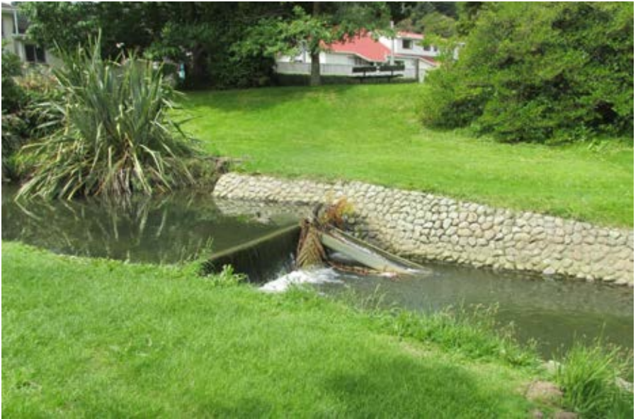
Fig. 2: St Ronans Avenue weir with floating fish ramp (note the use of the ramp by the local avian life)
